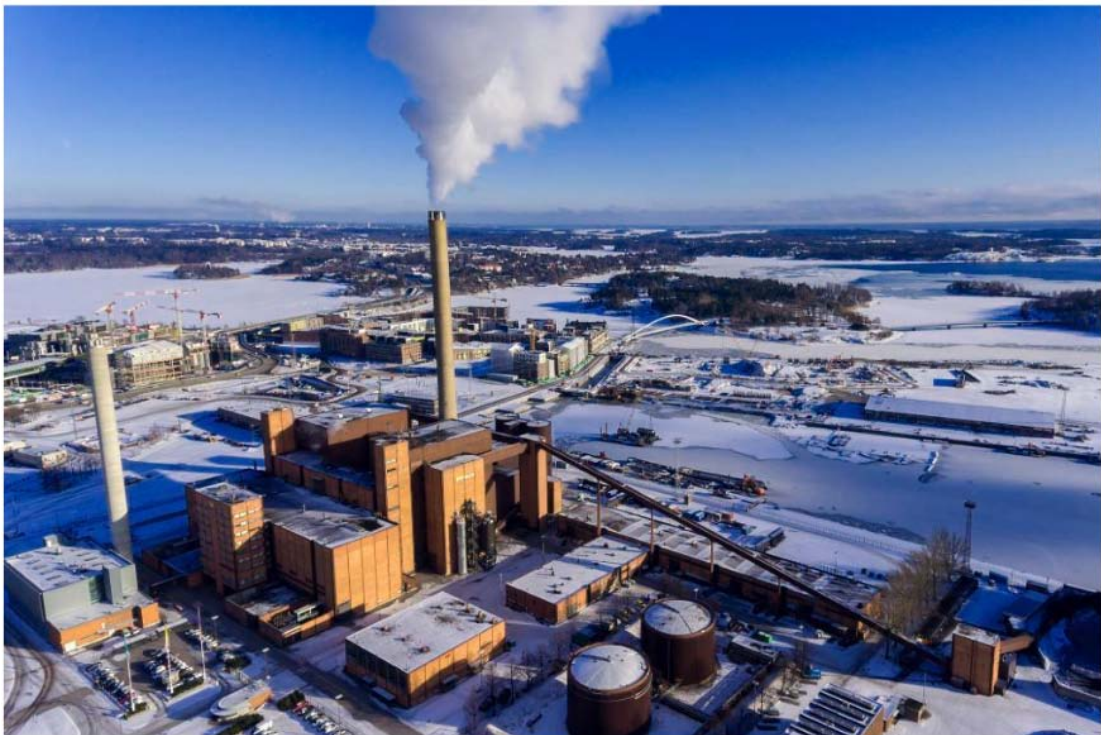
Figure 3: Hanasaari power station.
